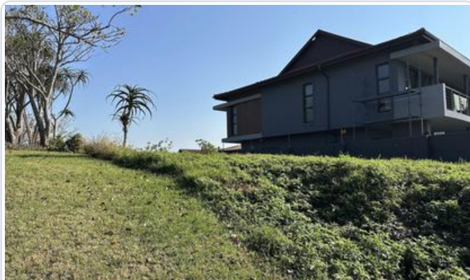
Existing neighbouring structure and slope
