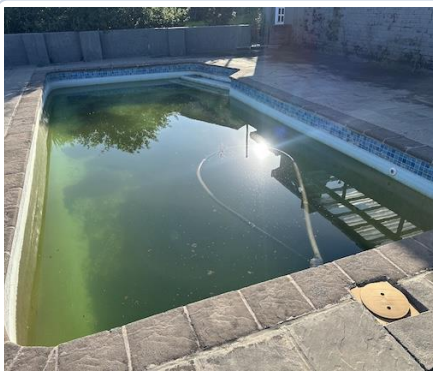
Swimming pool at inspection
