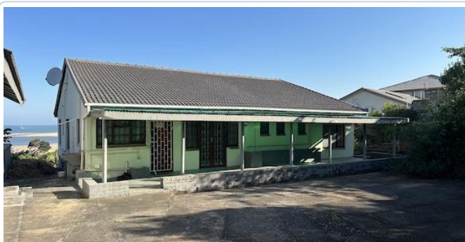
Main dwelling and paved forecourt
